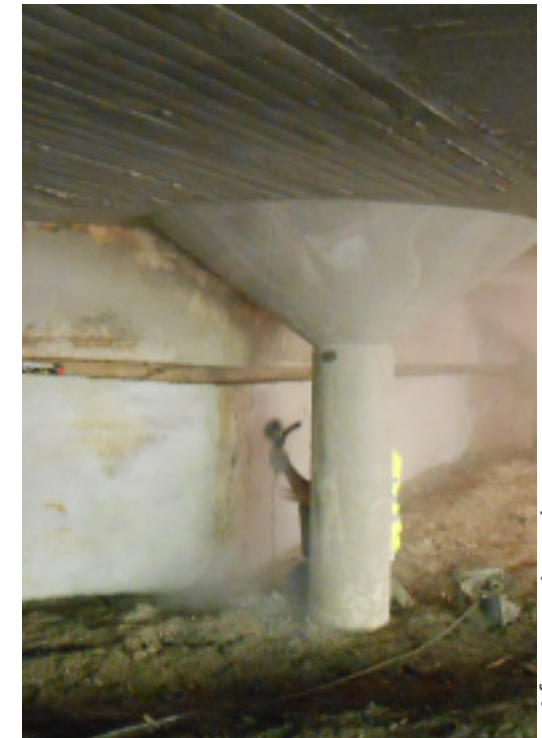
After repair actions
