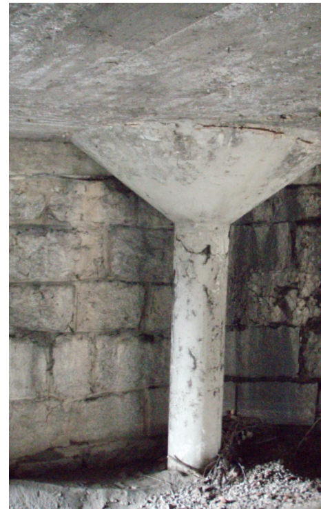
Before repair actions
