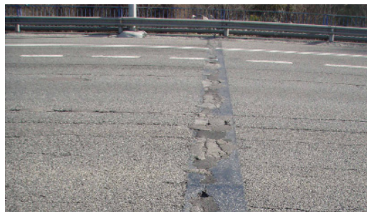
Before repair actions
