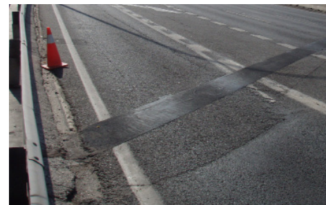
After repair actions
